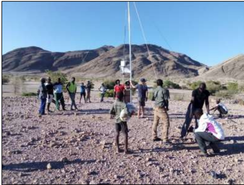
Early Warning Tower being erected
